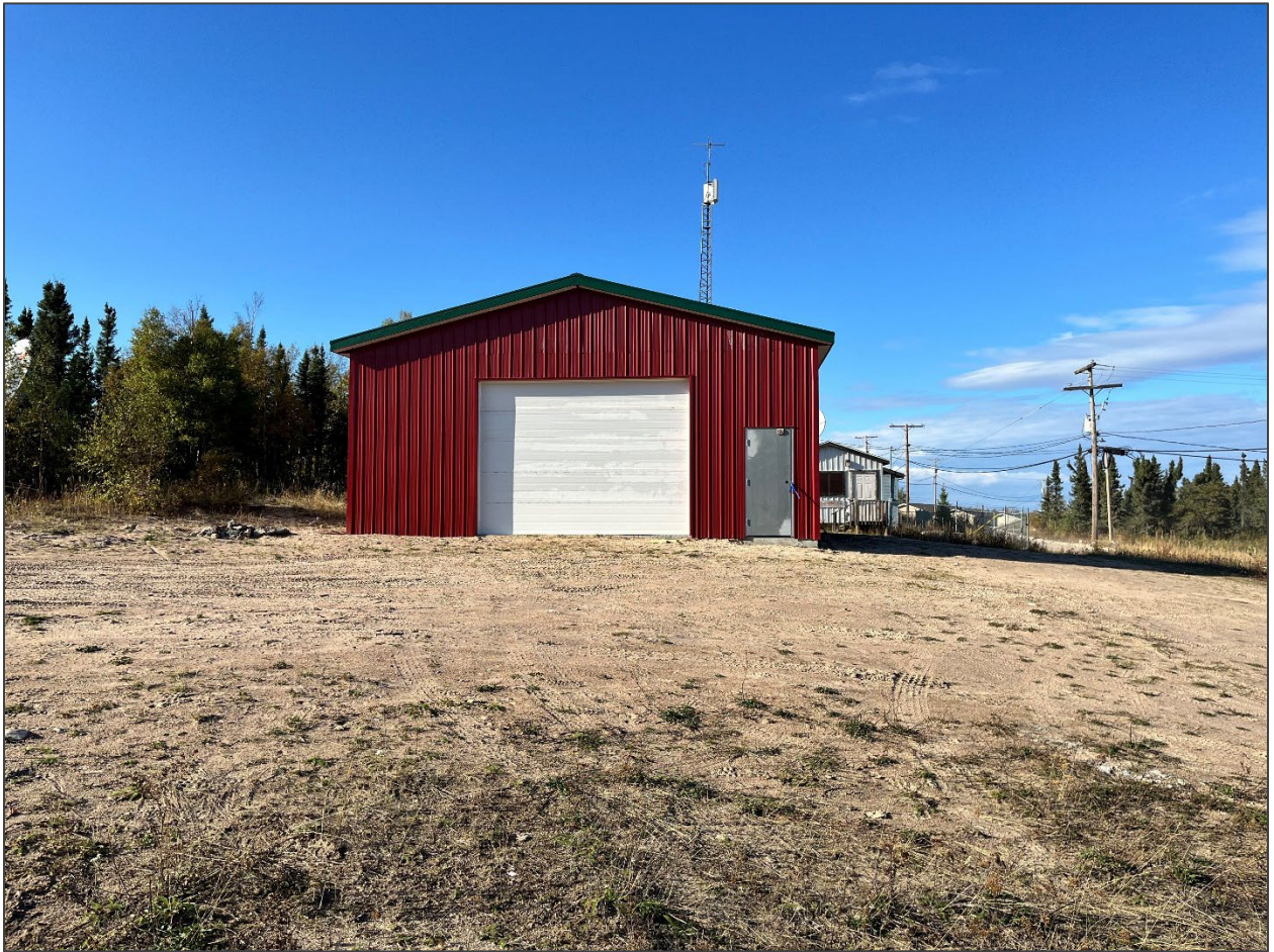
Picture 1: Front of Garage
